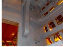
Below left Mark (he is abusy little bee isn't he?) has started making inroads into the hull up forward through a series of access hatchways cut through the moulds, Steve D is scarfing the very last timber for the Port side and far right Sadfie has started to fit some strengthening infills along the full length of the sheer
