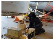
Below left John C is caulking the seam with caulking hammer to hand, middle Barnaby is working with Fay as she is burning off the old filler and paint in the area that we will be glass sheathing and over right below Sadie is also caulking the seam.
