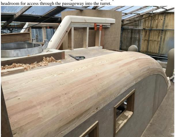
The shape is challenging as it rounds from sides to the top, and forward to aft, at the same time diminishing in width as the structure narrows towards the after deck.
