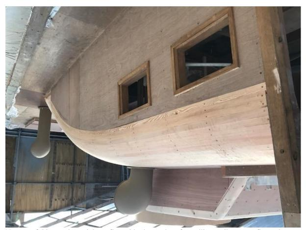
No part of this area is straight or flat, with plywood roof panelling scribe-cut to fit neatly around the turret which is just over one metre in diameter. The turret shown is a template made of hardboard, fitted to precisely match the Vickers Mark V design. The new turret is fabricated in aluminium and will be lifted into place next week.
