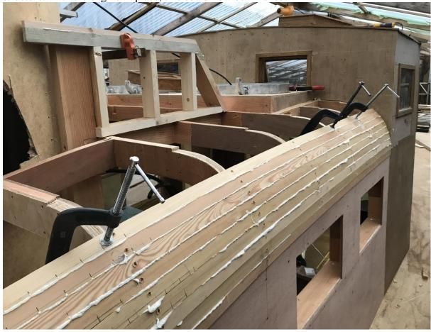
Sides have been clad in 12mm marine plywood. The rounded 'shoulders' were formed using larch battens - 14 lengths on each side, bent from the wheelhouse down to the after deck. The
